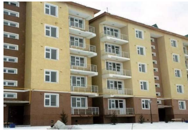
Location: Shymkent city, mcr.dstr. Asar Total area: 29580 sq.m Number of apartments: 522 Commissioned on: 14.09.2016, 19.09.2016, 20.09.2016
