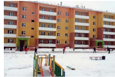
Location: Uralsk city, Zhachagansk town, mcr.dstr. Koktem Total area: 25166.5 sq.m Number of apartments: 500 Commissioned on: 21.12.2016
